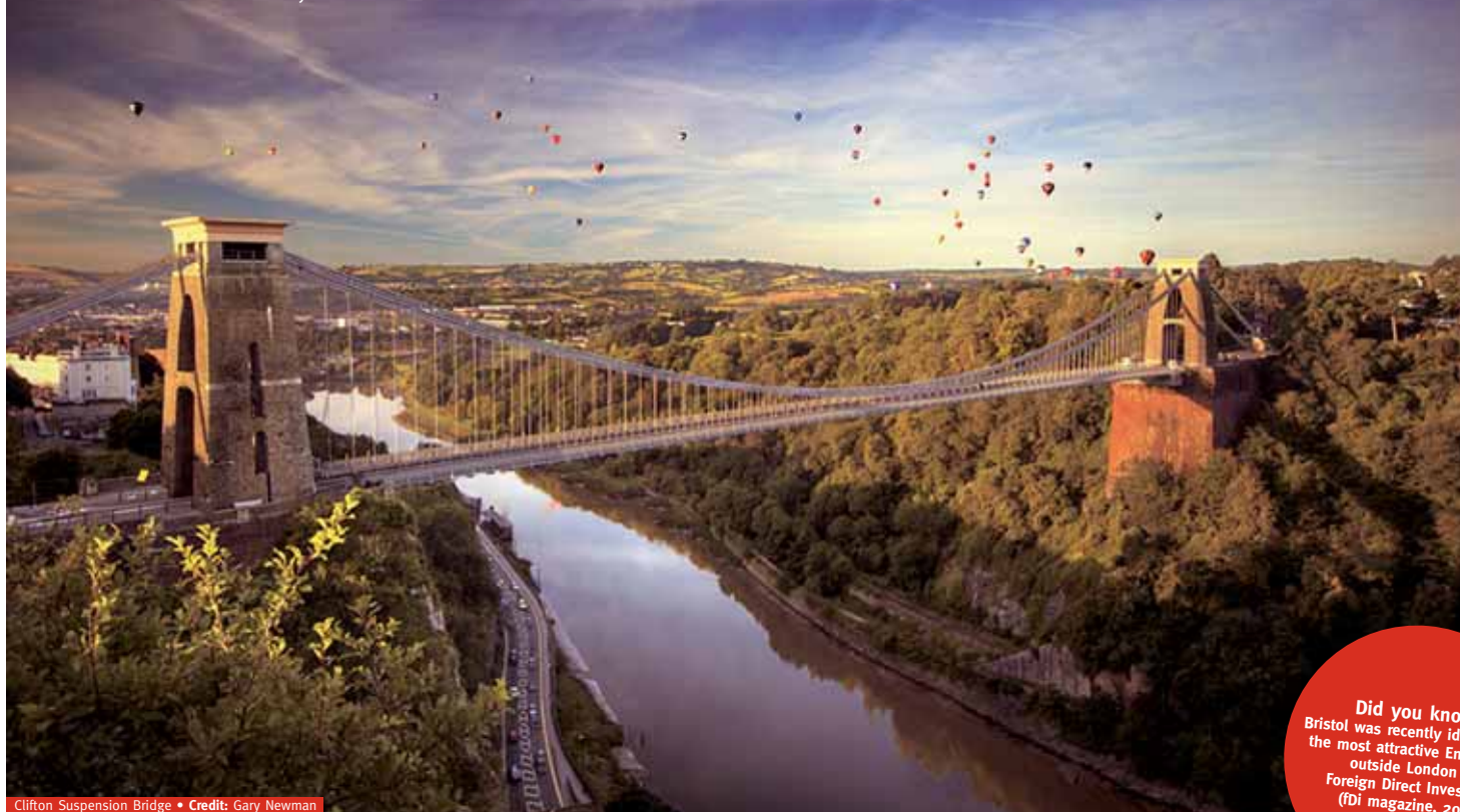
Clifton Suspension Bridge • Credit: Gary Newman
